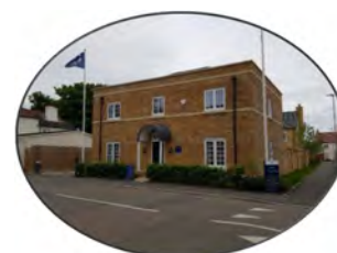
The Park new build along the High Street
