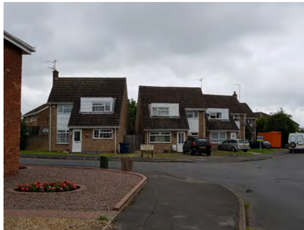
Properties with steeply pitched roofs on Pheasant Way
