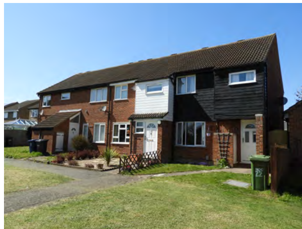
Dark and white weatherboarding provides distinct identity to homes in Kent Close
