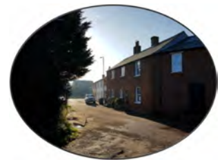
Terraces along Hardwick Lane with A1 access
