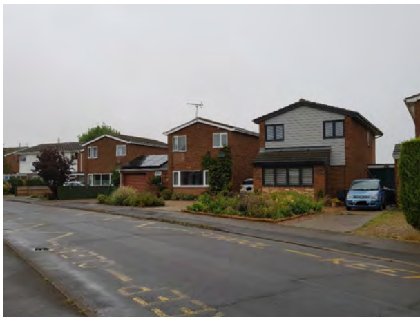
Detached homes along Humberdale Way, some have been extended and altered with new weatherboards
