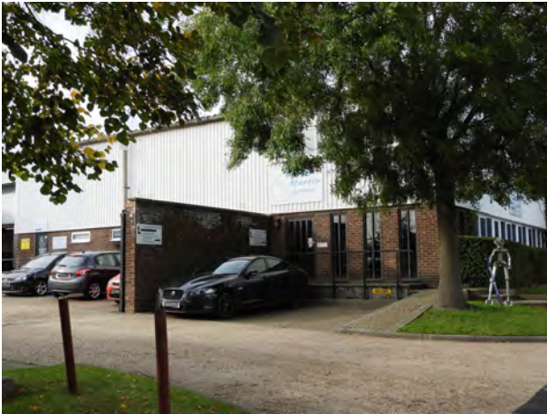
Brick buildings with clad upper elements are widespread in the industrial estates; this example contains a characterful piece of street art adding to a local sense of identity
