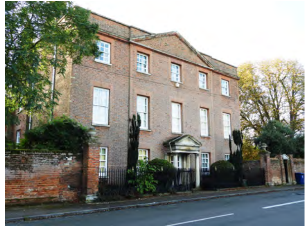
Built in 1746 Farm Hall presents a grand symmetrical frontage to West Street with the extensive gardens screened by soft red brick walling
