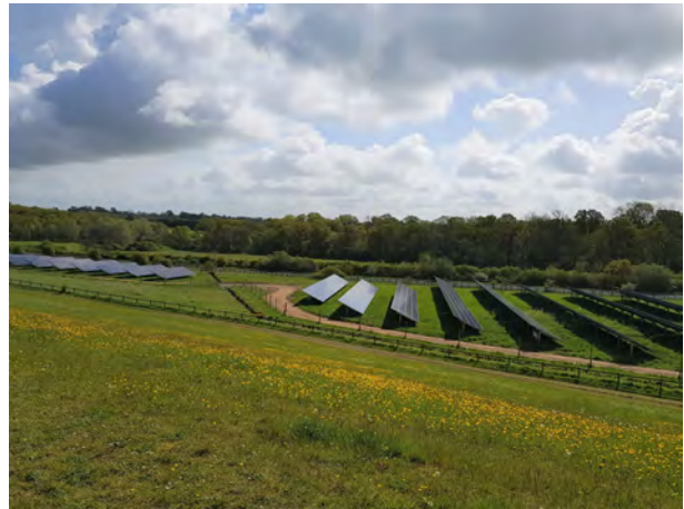
Solar panels south of Marlow Park
