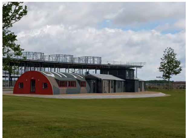
Former watch office/tower from Alconbury Airfield, recently refurbished as part of the redevelopment of the airfield
