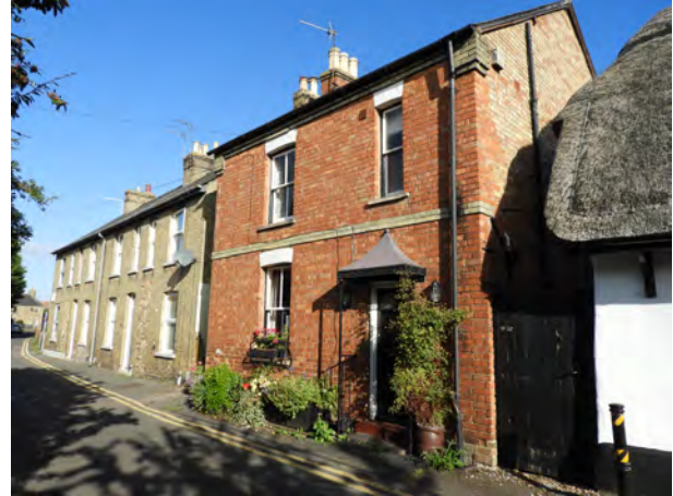
St Ann's Lane contains typical Victorian homes using a combination of buff and red brick
