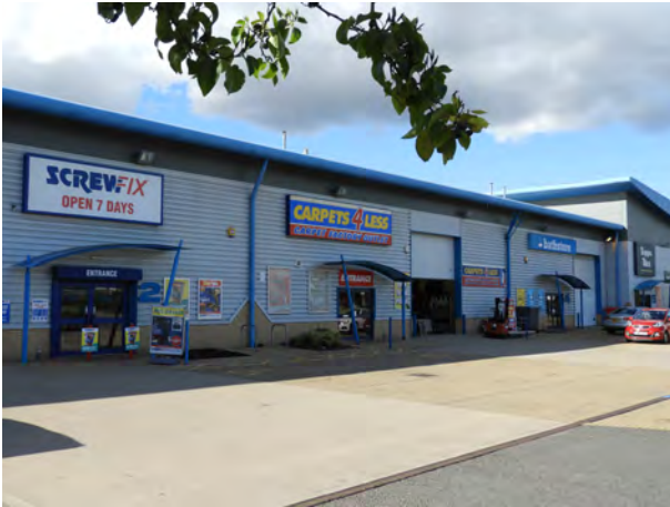
Bridge Centre, St Peter's Road - mixed industrial and trade counters
