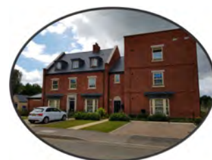
Further examples of house types, design and materials along Central Avenue
