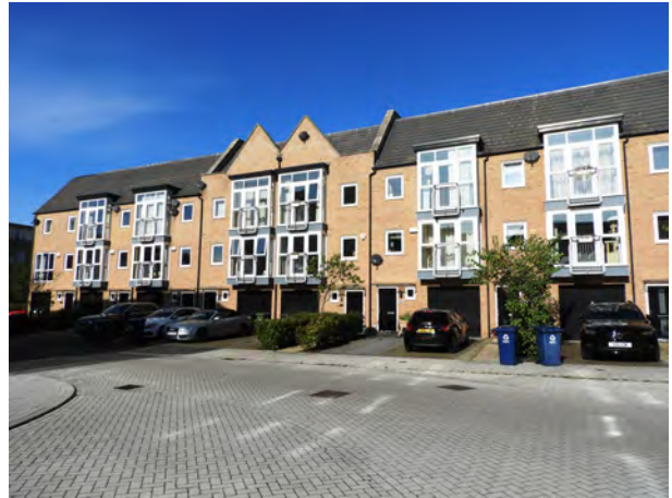
The three storey townhouses are typical of the increased focus in the early 21st century of making more efficient use of previously developed land
