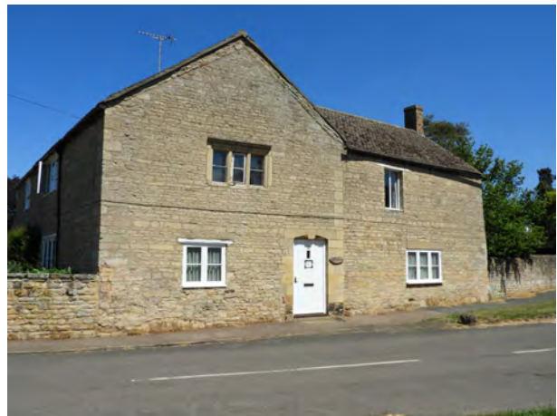
Old Mill House in Elton typifies the use of limestone and Collyweston slates of older buildings in the area
