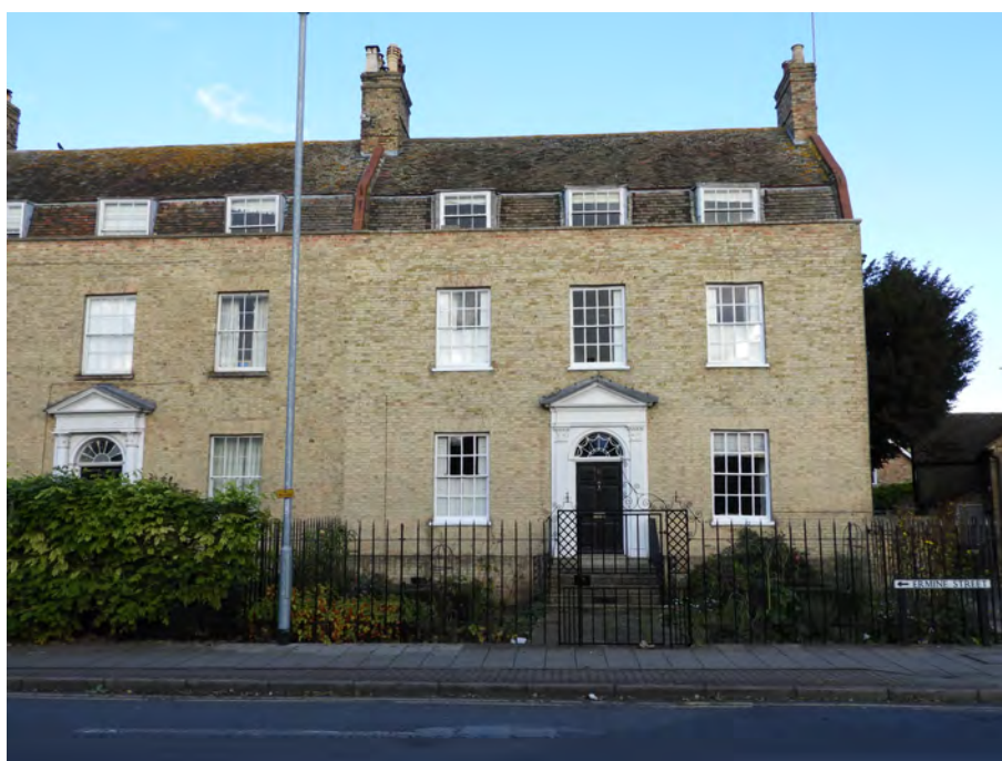
Late 18th Century gault brick town house at 79 Ermine Street, Huntingdon
