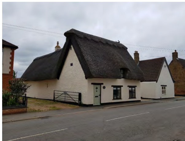
197 Main Street is an example of a thatched vernacular cottage
