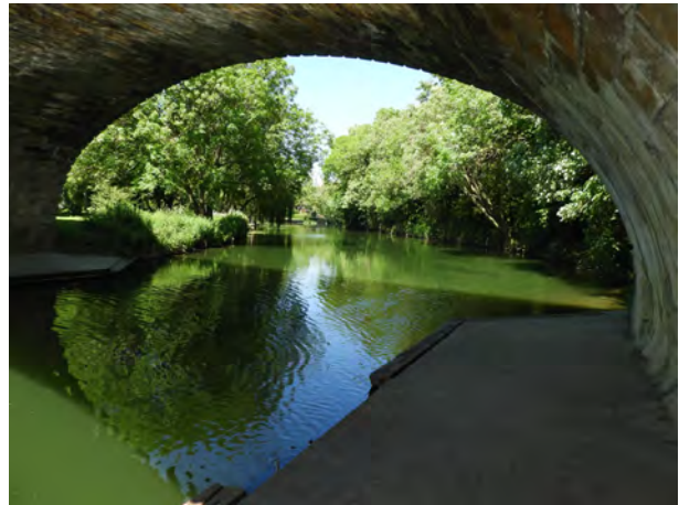
River Nene under the bridge at Wansford
