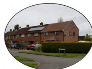
New build on Mandeville Road
