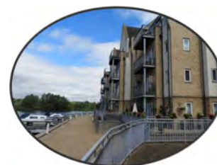
Apartments by moorings
