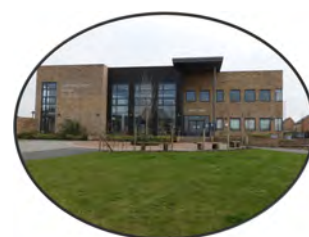
Godmanchester Bridge Academy
