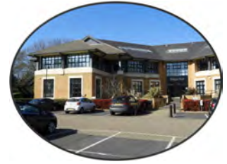
Offices at Parsons Green
