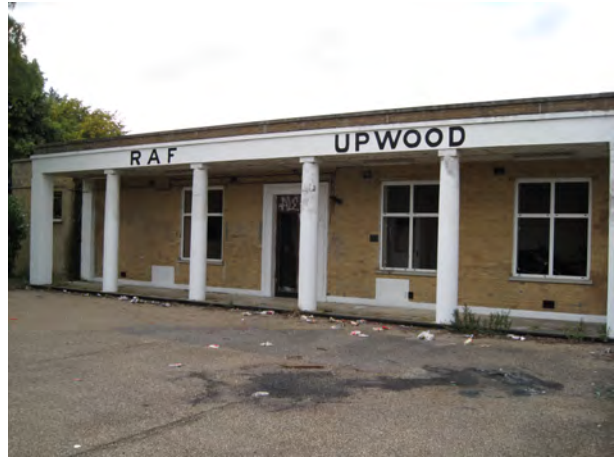
RAF Upwood contains a wide range of former military buildings, mostly of utilitarian architecture, vandalism and decay are damaging the historic character of the site
