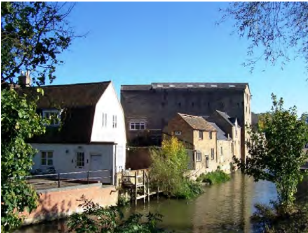
Buildings fronting onto Hen Brook reflect their historic waterfront uses
