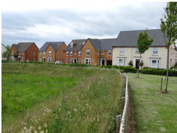
Homes within phase 1 of development along Collings Close facing onto a balancing pond
