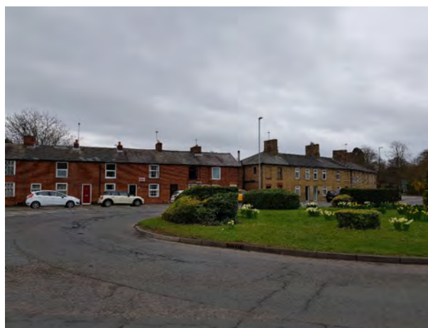
Terraces along Huntingdon Road facing onto the roundabout between Huntingdon Road, Church Road and Thrapston Road
