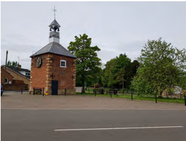
The listed Clock Tower and Lock-UP forms a focal point to the village and a memorable approach into the village from Huntingdon Road
