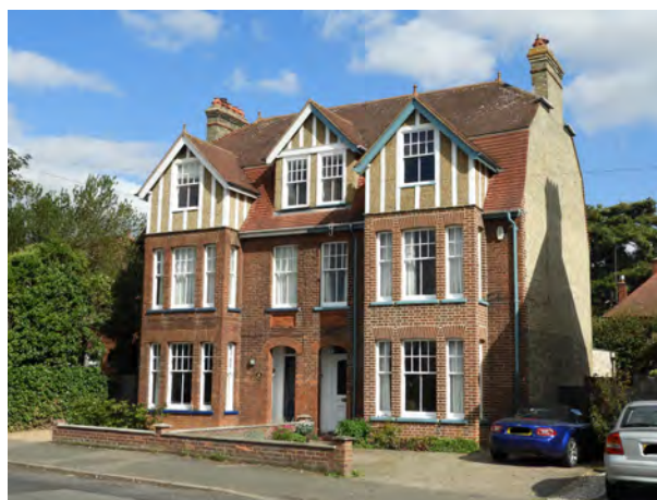
Victorian semi-detached villas, Needingworth Road, St Ives
