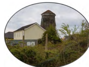
Mill Cottage and the Old Mill
