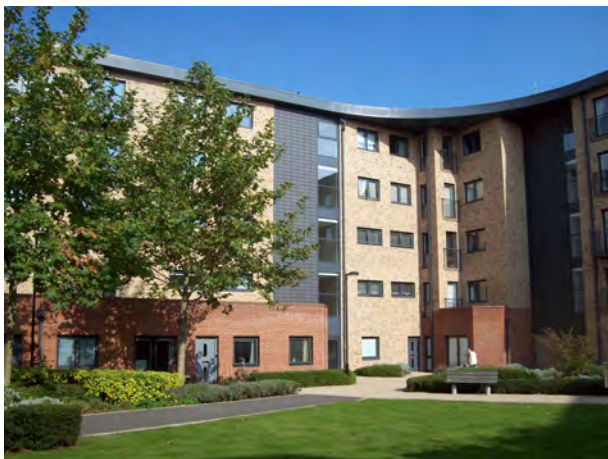
Hawkin's Court, Walden Road - high density town centre apartments utilising undercroft car parking to reduce the impact of parking on the streetscene
