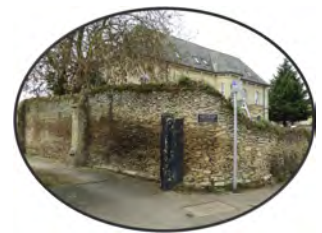
Priory barn walls
