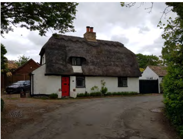
There are several cottages found within Fenstanton, some have thatched roofs
